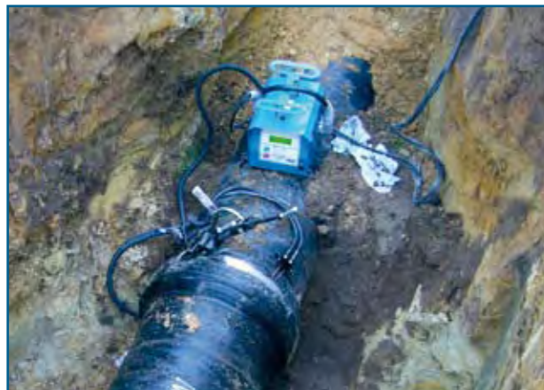
Electro fusion welding
