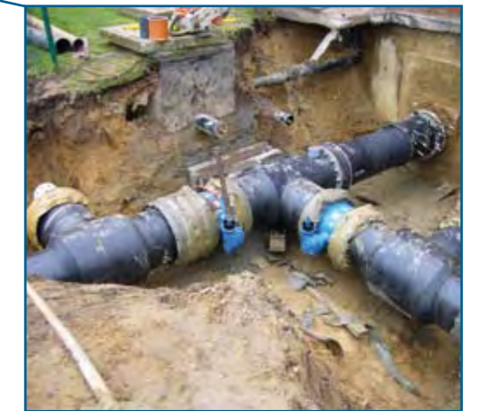
Distribution point - Connected T-pieces
