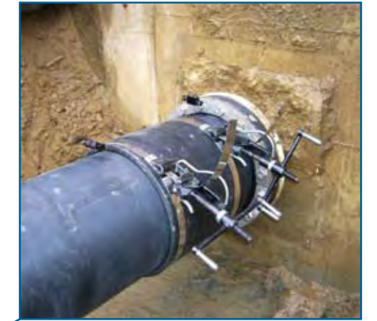
Slip-on socket with two integrated electro fusion joints
