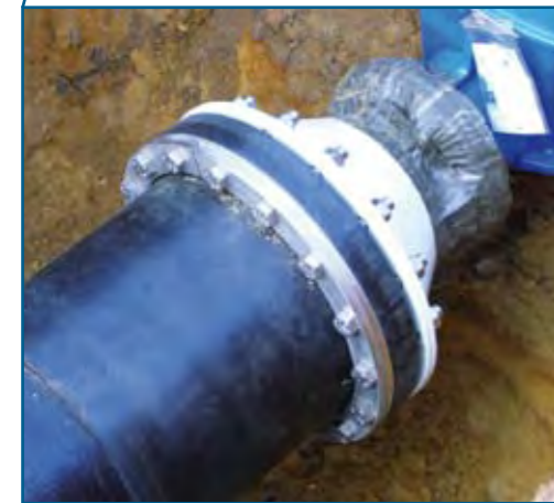
Flange connection to water pump station
