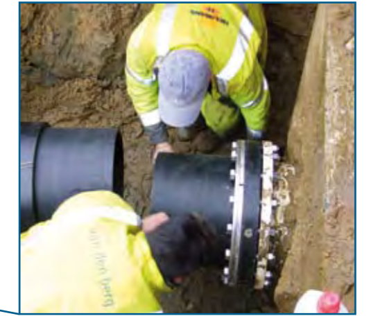
Wall connection (flange)
